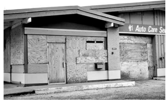
Under a new Village ordinance, vacant buildings such as this former Shell Station can no longer be boarded up.
